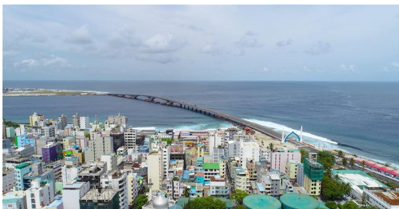
View of China-Maldives Friendship Bridge
